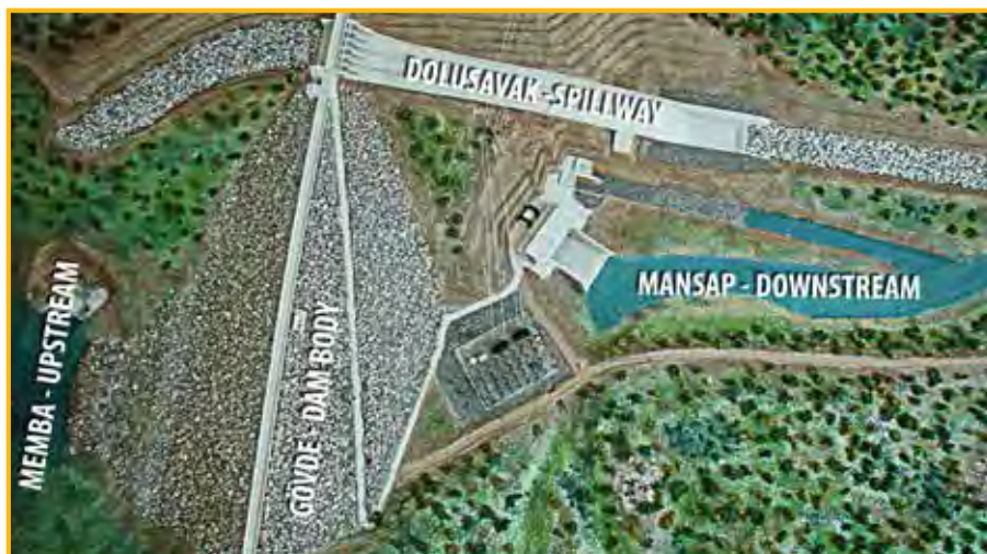
Figure 3: Model of Alpaslan II Dam and Spillway on the Murat River
